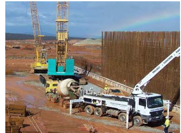
Boddington mine under construction
